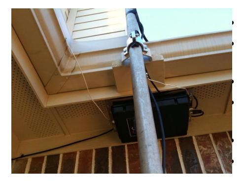
Should be a new gutter May required sections to be bonded together The longer the better Gutter & Downspouts can't be grounded Ground and radials required Remote tuner required
